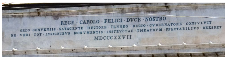
Figure 2.1: Close up of the top of Galleria Giuseppe Siri
